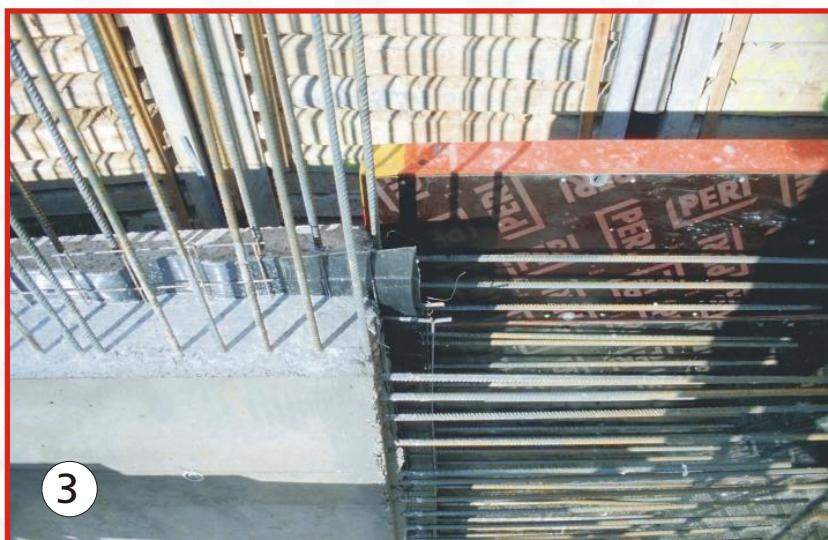
The photos show an old design in which the joint band was held by a constructional steel mat (1, 2, 3).
