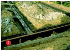
MSL - girder casing system Type FS-U-Shaped
