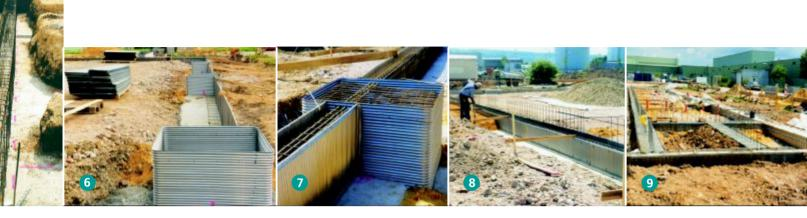
Formed pieces, e.g. angled elements (Photo 17), are produced quickly and easily by cutting into the cross-sections and bending to the required position on site.
