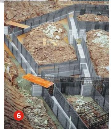
Corners can easily be made by the client by cutting and tying with wire on site. Photos 1, 3 and 4 show a building section with shuttering partially filled with concrete, soil or still freestanding.
