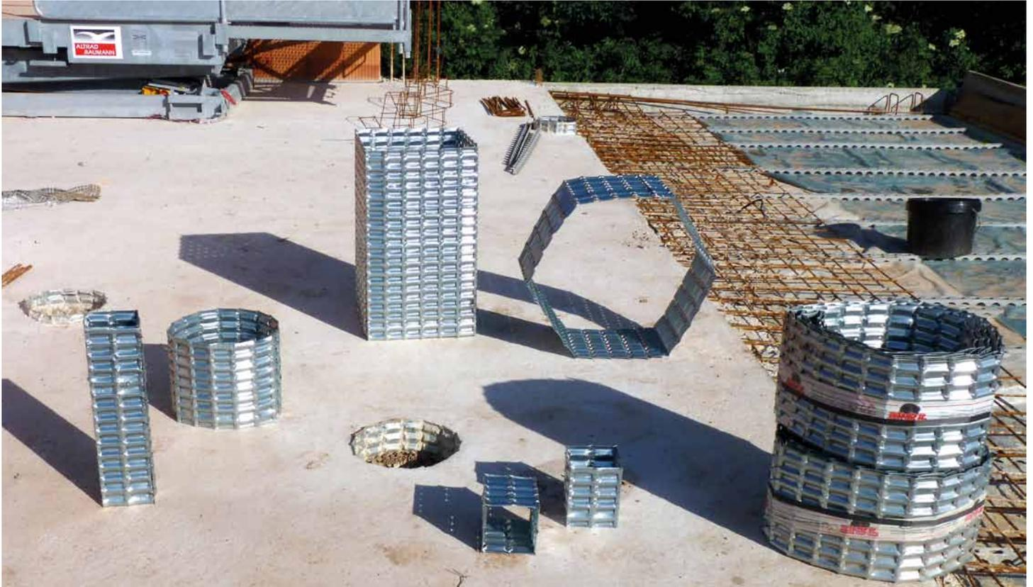
The MSL cavity system Vario is offered in widths from 130 mm to 890 mm as rolled materials with 6 m formwork length.
